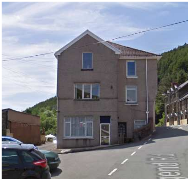
Figure 3 – Front elevation of 1/1A Chapel Street
